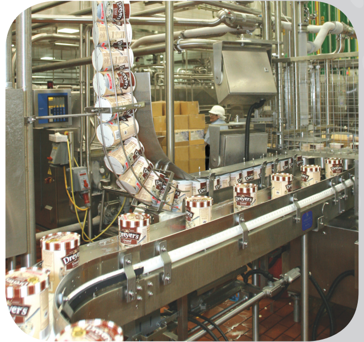
Nercon's engineering team provides packaging line layouts, line efficiency studies, project management, mechanical and electrical engineering, installation and site management.
