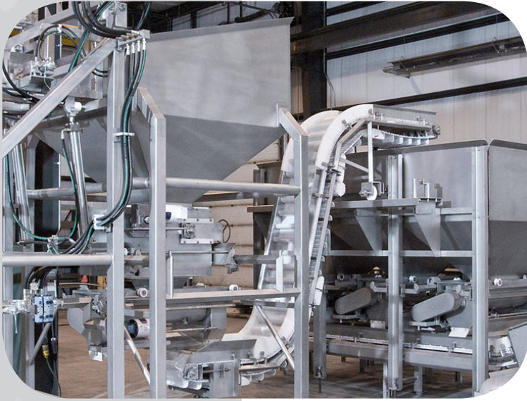
Hopper Conveyor System
